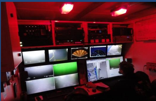
ROV CONTROL CABIN
